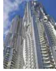
Structural Design of the Year, 8 Spruce Street-Beekman Tower
